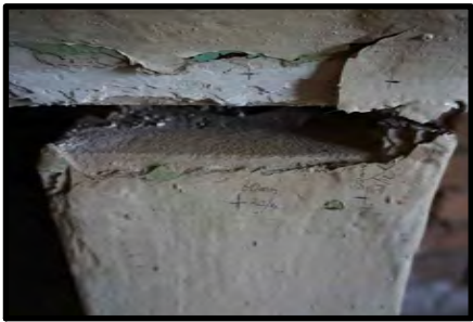
06 DETAIL IMAGES -- OPENING JOINTS OF CHIMNEY PIECE, 2019 NORTHERN WALL
