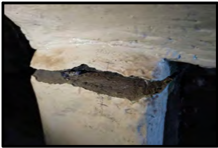
06 DETAIL IMAGES -- OPENING JOINTS OF CHIMNEY PIECE, 2019 NORTHERN WALL
